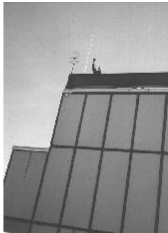
Fig. 10.11 Roof-top site contracts have value in a facilities sale
