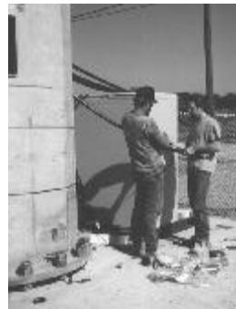
Fig.10.16 Be ready to replace transmission lines for a nice business
